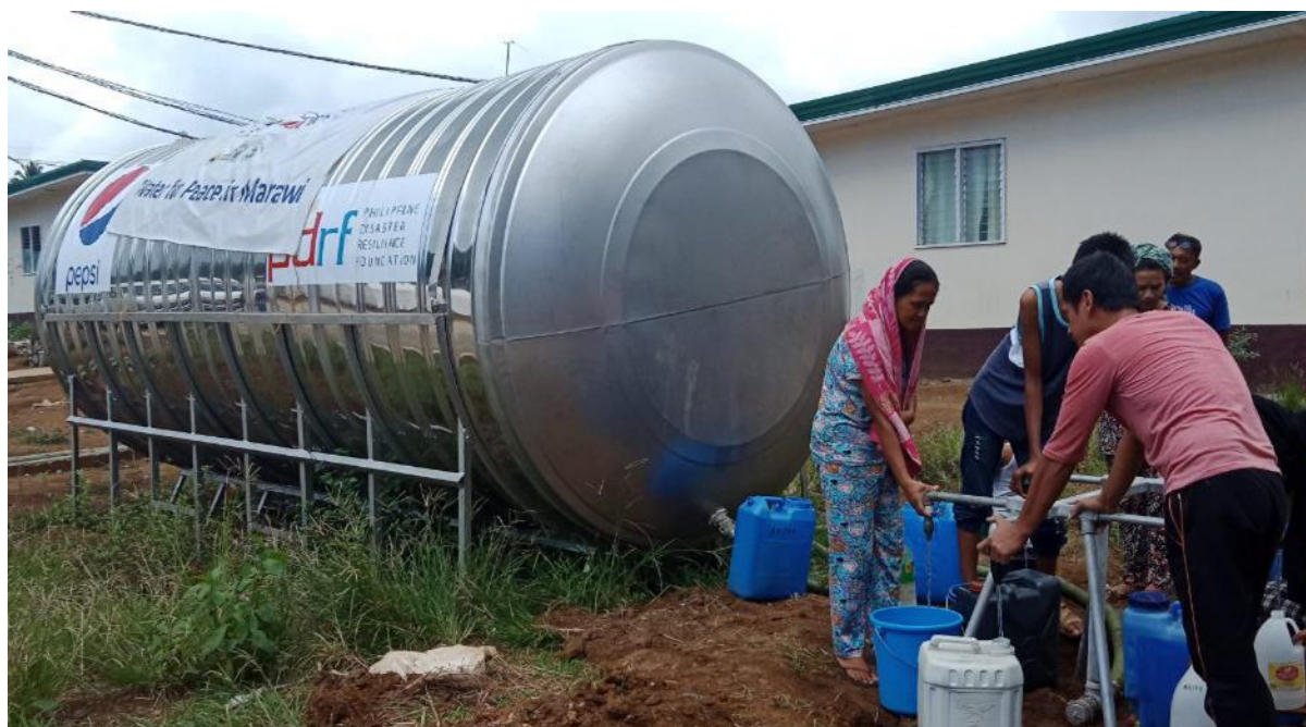
PDRF installed 50,000-liter water tanks in Marawi City in partnership with Pepsi-Cola Products. Photo: PDRF
